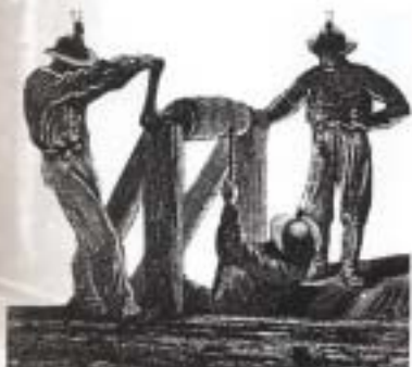
Hand winding gear used to lower men into the shafts
