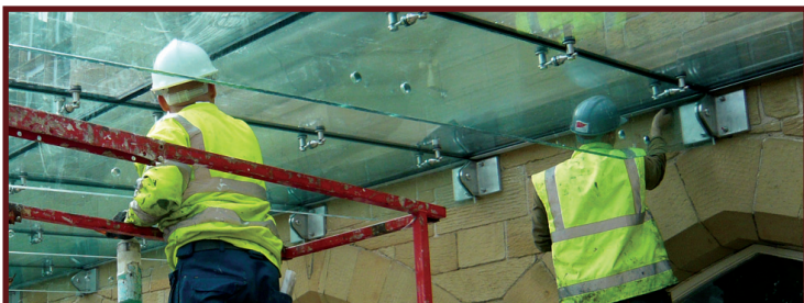
Ensuring the glazed extension is watertight.
