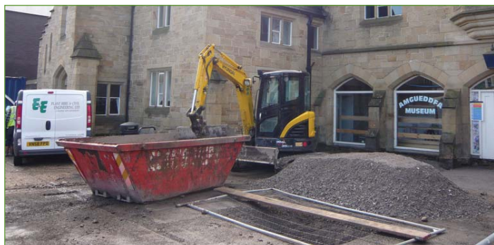
Preparing the foundations for the new glazed extension
