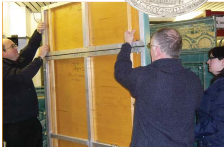
Carefully dismantling the tiled porch to go into storage
