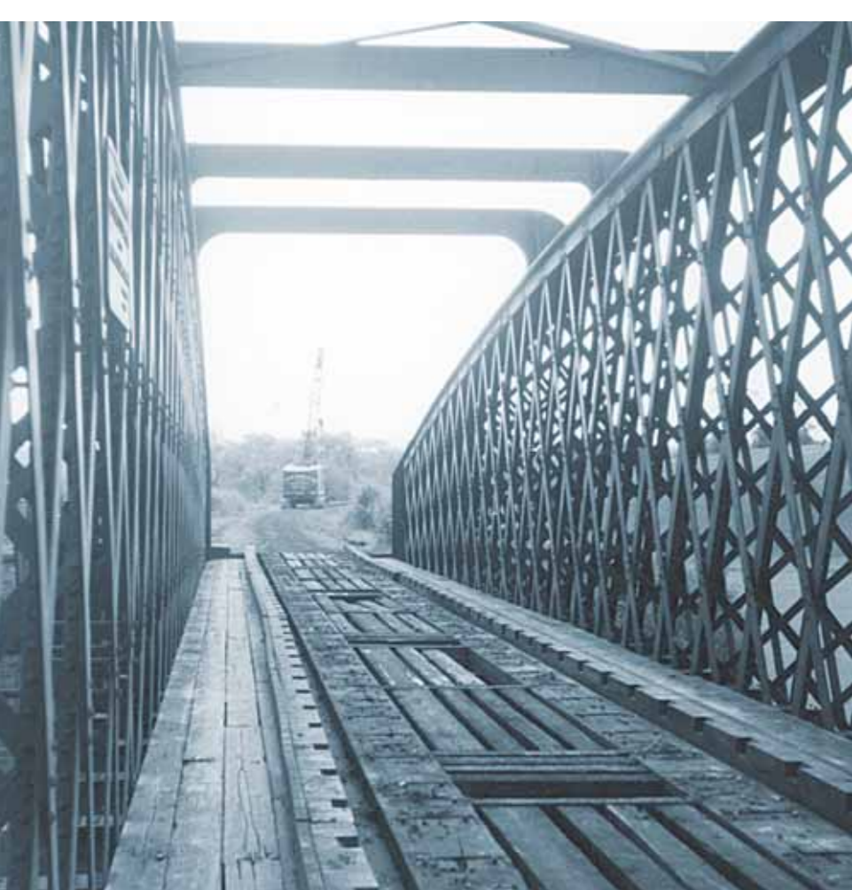
The Iron Bridge - the railway bridge over the River Dee Y Bont Haearn - y bont reilffordd dros yr afon Dyfrdwy
