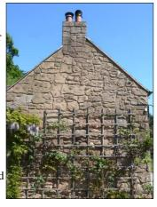
and texture and historically would have consisted of lime and sand. Modern hard cement mortar and renders prevent the evaporation of moisture which can accumulate within the wall causing damp internally. When appropriate, hard cement renders should be replaced with a lime alternative.
