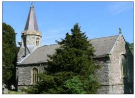
style with segmental pointed heads. The three-stage west tower supports a short slate covered spire with weathervane atop. Internally, the Church comprises a single chamber nave and chancel with a five bay roof constructed of collar trusses supported by straight braces.
