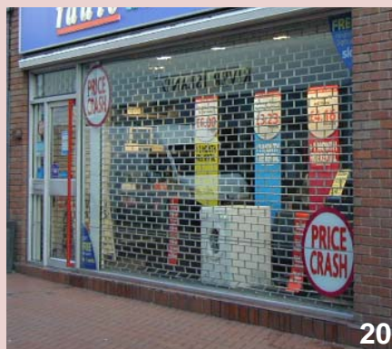
20 & 21. Internally fitted shutters and grilles are less visually intrusive.
