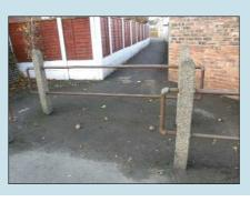
are in a poor condition with much of the concrete eroded and the metal rails rusting which detract from the general appearance of the streetscape. The modern concrete is an appropriate material for the Conservation Area and the replacement of the bollards and rails with a more traditional cast iron structure would significantly enhance the appearance of the street and the setting of the Conservation Area when arriving from Piercy Avenue.
